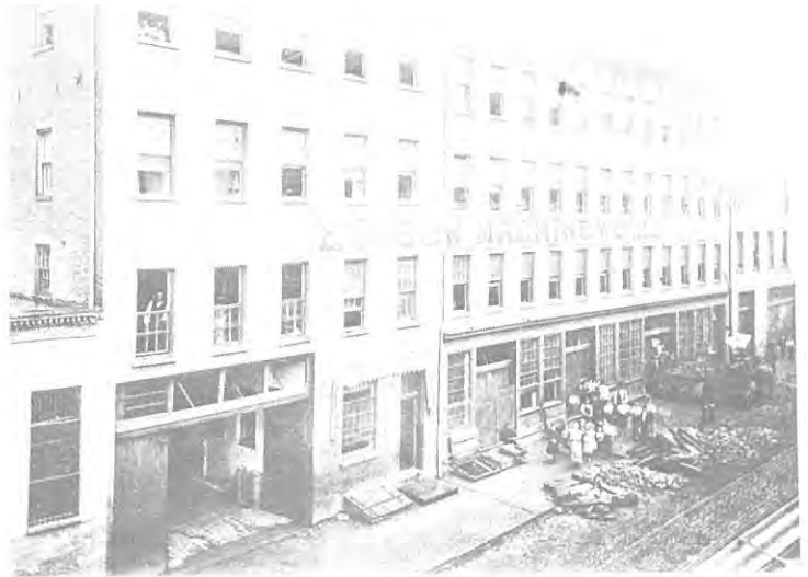
The Edison Machine Works, Goerck Street, New York City.
